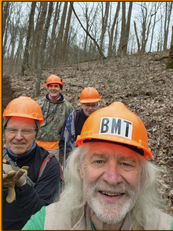
Andy Meeks, Ian Guttridge, Steve Dennison and David Watkins teamed up to work on sidehilling a steep section of 12b. This was a tough stretch for a crew of four but they were able to dig out 1200 feet of trail.
