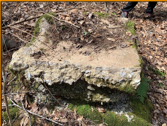
Due to the pipe that protruded from it, folks thought this structure was either a shower base or a toilet base.
