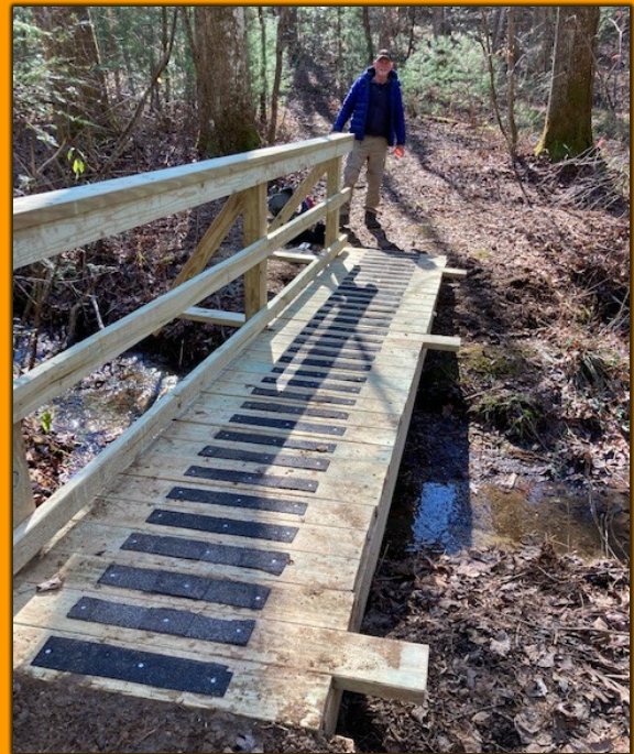
Mill Creek Bridge!!
