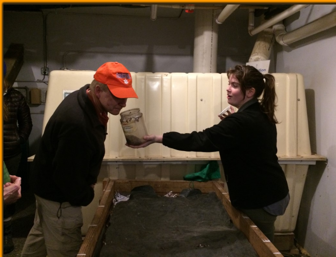
Our five o'clock tour included the worm beds and toilet composting facility. The Hike Inn achieved LEED Platinum status level in 2019.
