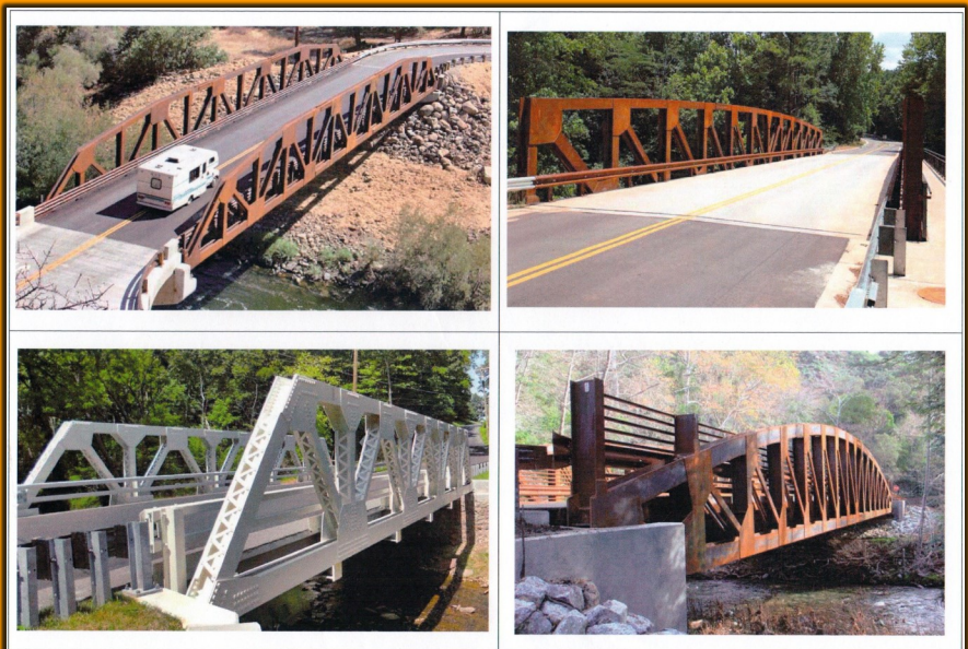
EXAMPLE TRUSS BRIDGES
