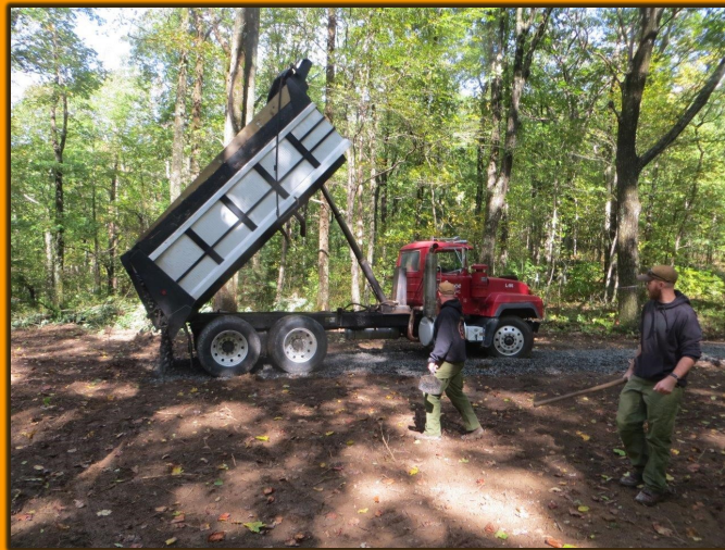
Gravel begins to be dumped.
