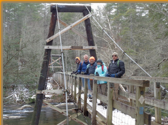
The footing was challenging! Inches of frozen ice!
