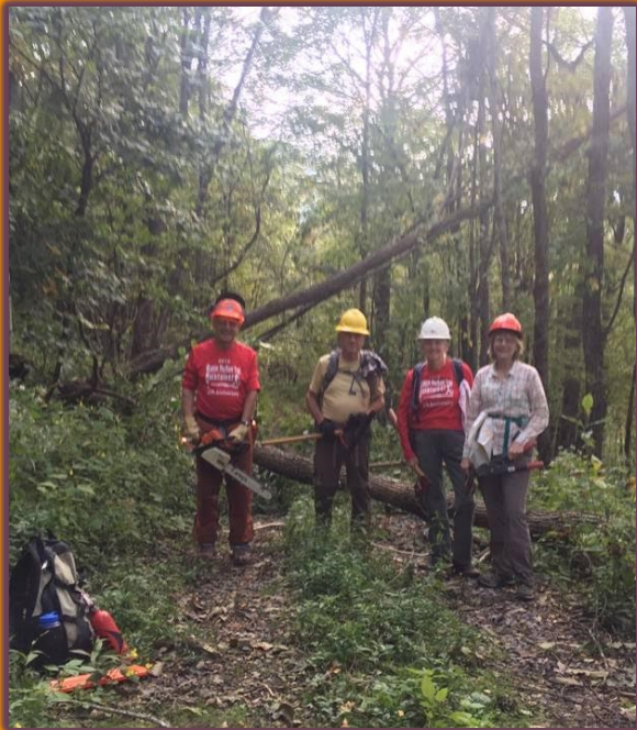
Work began right at the trailhead on the upper end.
