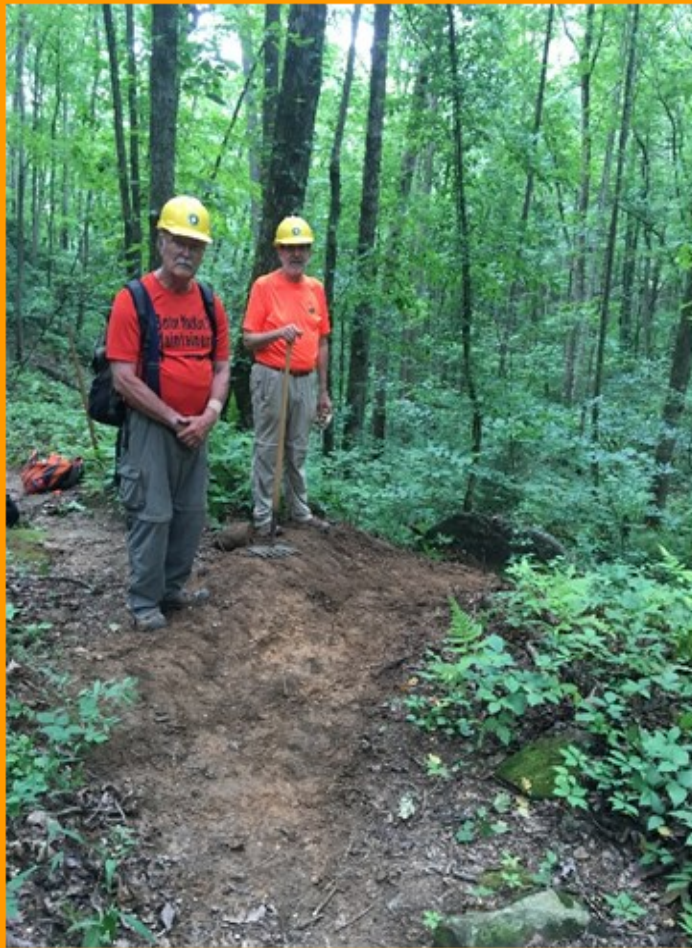
Ralph Heller and Ken Cissna preside over a fine specimen of a water diversion.
