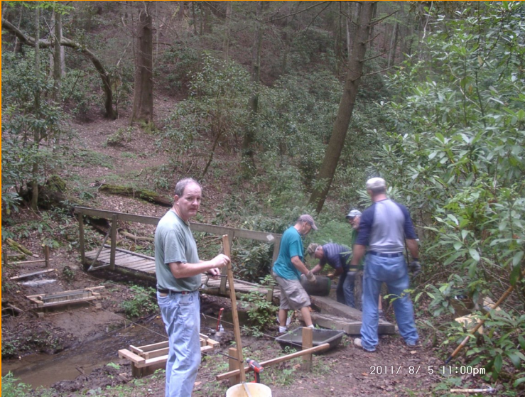
Marty Dominy supervising construction of bridge in 2011
