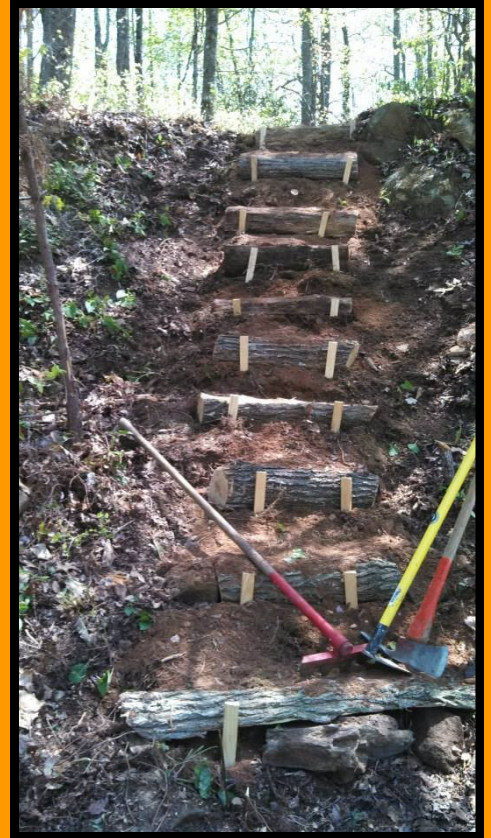
New Stair Construction
