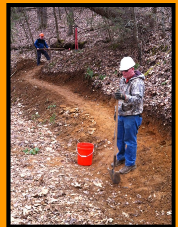
George Owen (back left) and Kyle Atkins finish the "Entrance Ramp."
