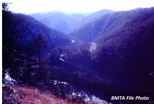
On the sharp ridge south of Ocoee #2 Dam looking west or downstream over the Ocoee River Gorge. It's doubtful you actually can see the river due to the shadows, but the highway is on the right and the flume is on the left. This was the ridge Clayton Pannell and Dominy descended.
