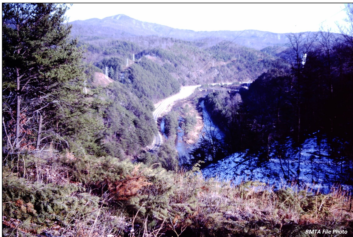
In this picture, you can see the powerlines, the highway, the river, the bridge over the river at Ocoee #3 Powerhouse, and if you look carefully, the surge tank above the powerhouse. The ridge in the background should be the south end of Little Frog Mountain with the high point on the left being Panther Knob
